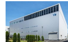
Fujisawa Plant New building for the development of semiconductor manufacturing equipment
