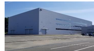
Kumamoto Plant New production building (K3)
