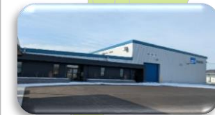
Ebara Field Tech Tohoku Plant
